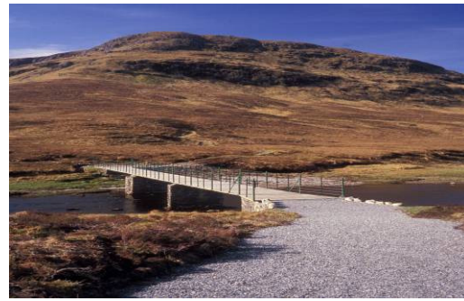
New footbridge over Abhainn Cuileig Photo: D Sime
